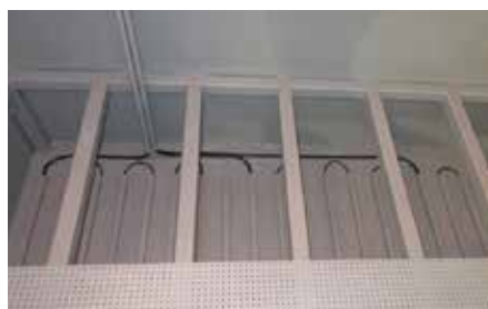
The GeoBag™ units can be isolated and heated for areas with colder climates.
